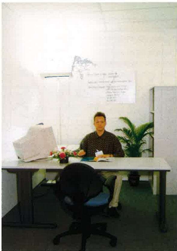
System 5. This used an Iguzzini Vela 2x36 watt uplight (with a downward component) and a Tavolo 1x11 watt task light from Relux Lighting (FE), Singapore.
