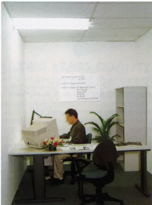
System 4. This used a Zumtobel RCE 2x32 watt (Mellowlight) luminaire supplied by Elite Manufacturing Co, Singapore. The task light was a Zumtobel OC-T 2x9 watt.
