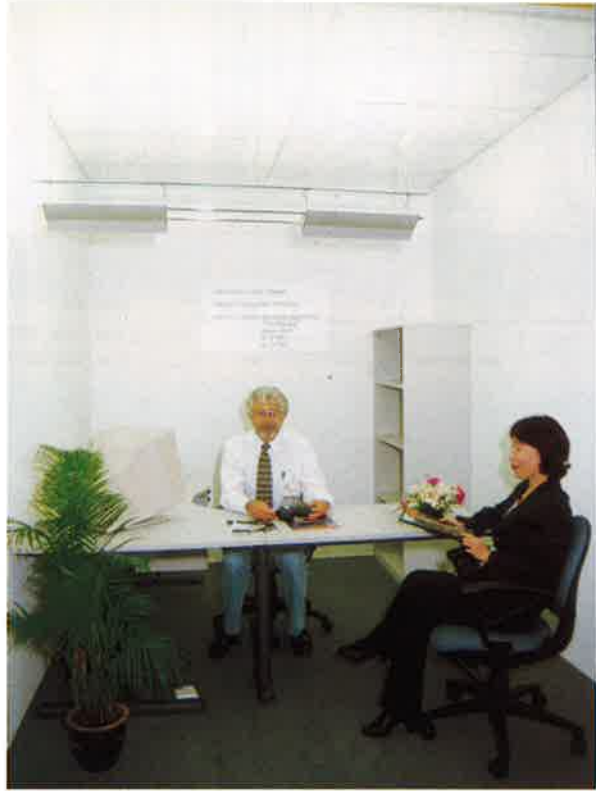
System 3. This used a Cosmolight 4x36 watt (TC-L) luminaire supplied by Thorn Lighting, Singapore.
